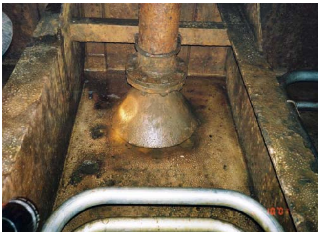
Bell-mouths in W.B.T. are considered critical locations for local wastage in all types of vessels
