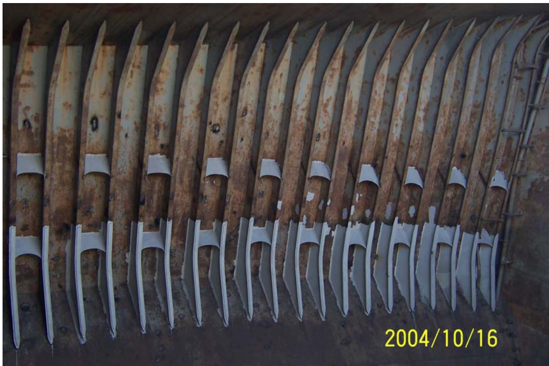
Above – structural reinforcement using Tripping Brackets
