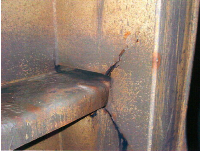
Thickness reductions, cracks & other defects can be easily identified after cleaning & removal of all loose accumulated corrosion scale
