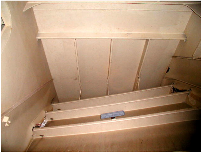
Lighting can reveal the full extent of defects, corrosion or deformations in a confined space
