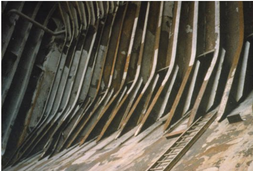
Unacceptable means of access to side shell frames of single skin bulk carriers via unsecured ladder
