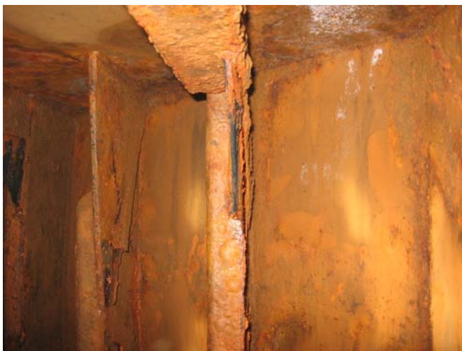
A typical stiffener & end bracket in a W.B.T. after chipping – cleaning may reveal the true thickness reduction it is subjected to
