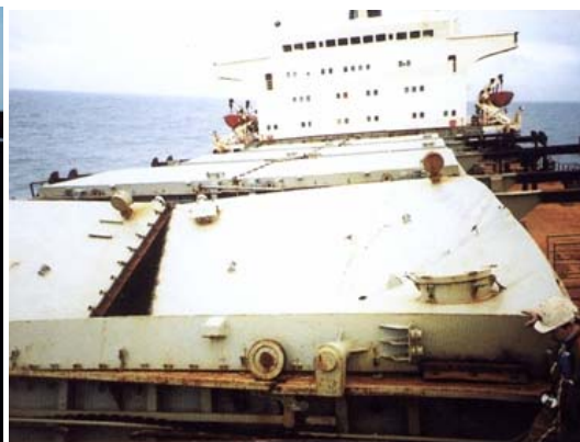
Catastrophic failure – collapsed hatch cover
